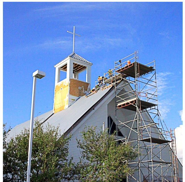
Finishing the bell tower
